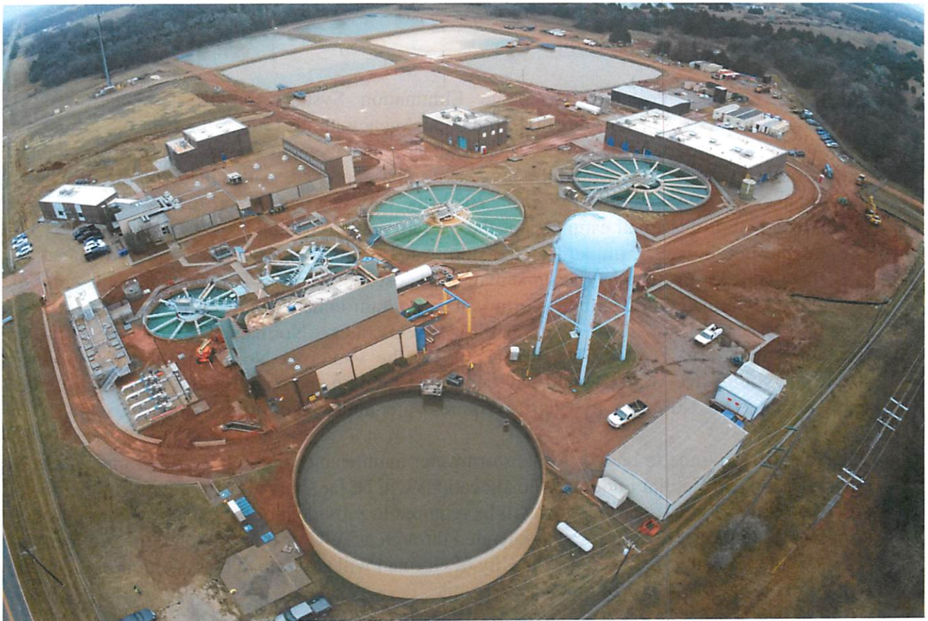
Improvements to Norman Water Treatment Plant
